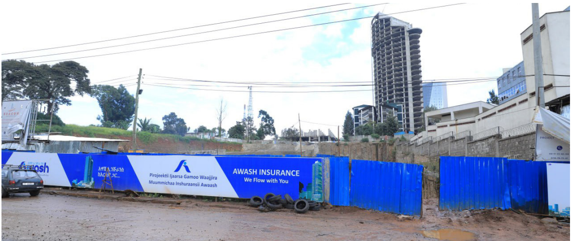
HQs Building shoring work
