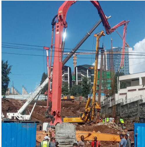
New HQs Shoring Work
